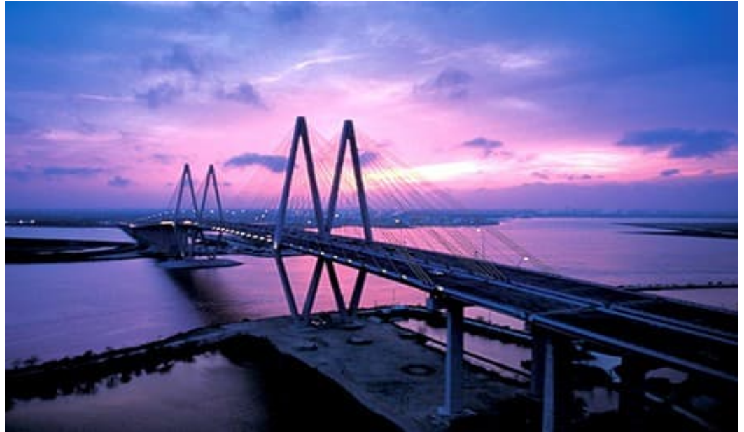
Fred Hartman Bridge – Baytown, TX
