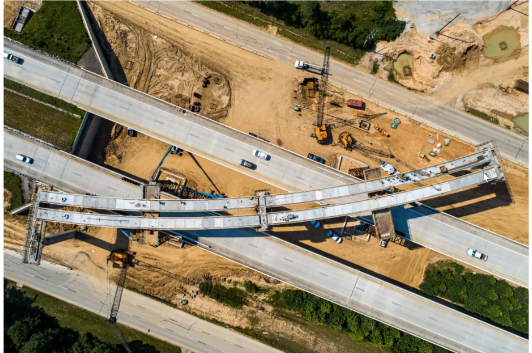
Aerial View of SH249/SH99 Intersection Bridge Under Construction
